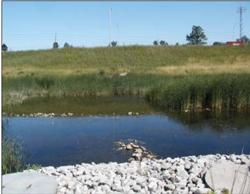
D6: Tributary of the East Don River, facing upstream (north) towards the Highway 7 culvert.
