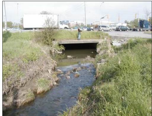
R15: Beaver Creek facing upstream (northwest) towards the Woodbine Avenue culvert.
