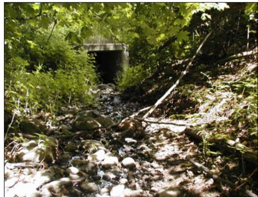
D22: Tributary of the East Don River, facing downstream (east) towards the Bathurst Street culvert.
