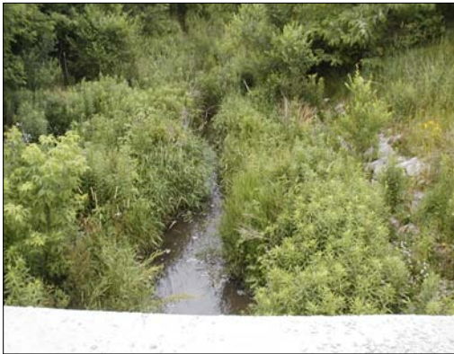
D8: Tributary of the East Don River, facing downstream (southeast) from the Highway 7/Yonge Street culvert.
