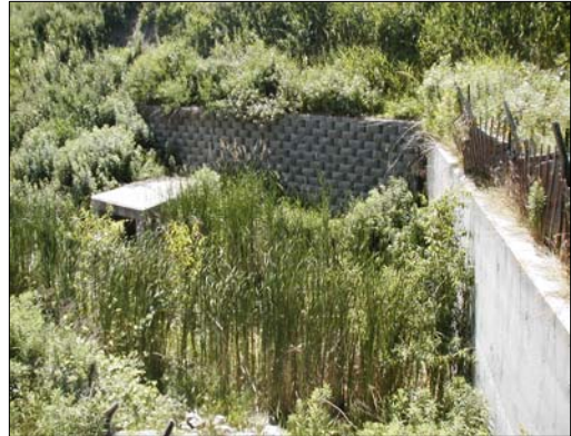
D22: Tributary of the East Don River, facing upstream (west) towards the Bathurst Street culvert.
