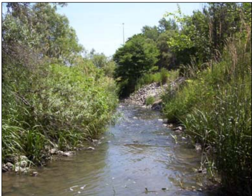
D12: German Mills Creek facing downstream (south) from the Highway 7 culvert.
