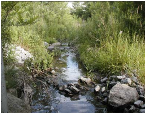
D9: Tributary of the East Don River, facing upstream (north) from the Highway 407/Langstaff Road culvert.
