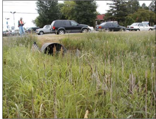
R22: Tributary of the Lower Rouge River, facing downstream (east) towards the Main Street Unionville culvert.
