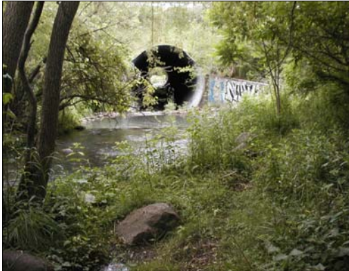
R8: Robinson Creek facing downstream (south) towards the Highway 7 culvert.
