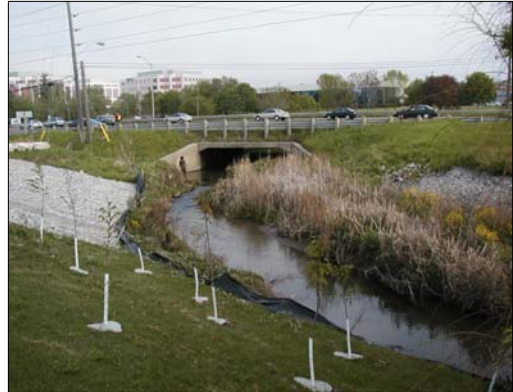
R2: Beaver Creek facing upstream (north) towards the Highway 7 culvert.
