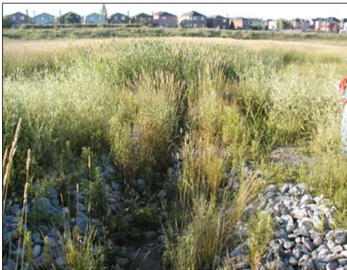
D18: Tributary of Westminister Creek facing downstream (south) from the culvert, south of Highway 407.
