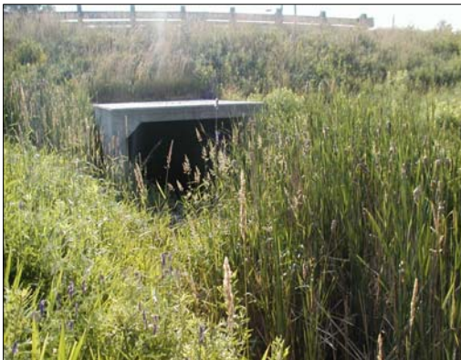
H14: Tributary of Black Creek, facing upstream (east) towards the Jane Street culvert.
