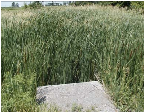
R13: Tributary of the Little Rouge River, facing upstream (north) from the Highway 7 culvert.
