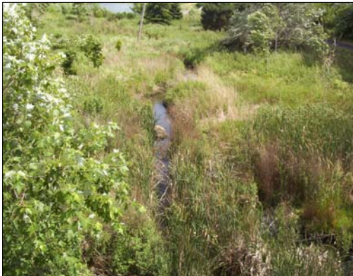
D14: Tributary of German Mills Creek, facing downstream (south) from the Highway 7 culvert.
