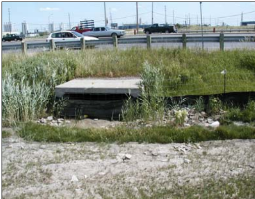
H4: Tributary of the Main Humber River, facing downstream (south) towards the Highway 7 culvert.
