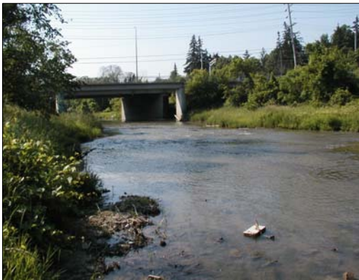
H7: The Main Humber River, facing downstream (south) towards the Highway 7 bridge.
