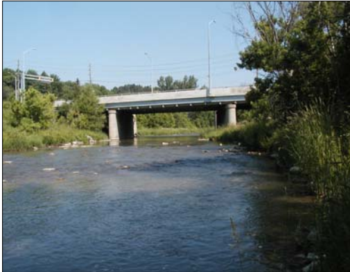
H7: The Main Humber River, facing upstream (north) towards the Highway 7 bridge.
