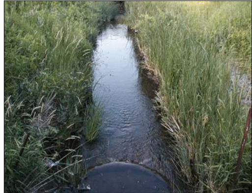
H12: Black Creek facing downstream (south) from the Highway 7 culvert.
