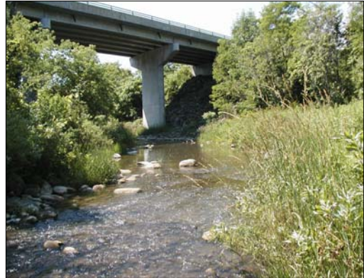
R14: The Little Rouge River facing downstream (south) towards the Highway 7 bridge.
