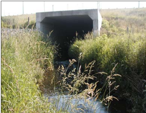
H12: Black Creek facing upstream (north) towards the Highway 7 culvert.
