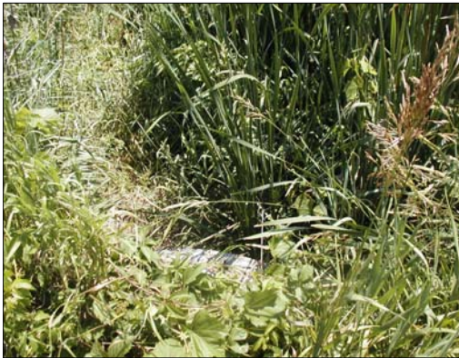
P1: Tributary of Petticoat Creek, facing downstream (south) from the Highway 7 culvert
