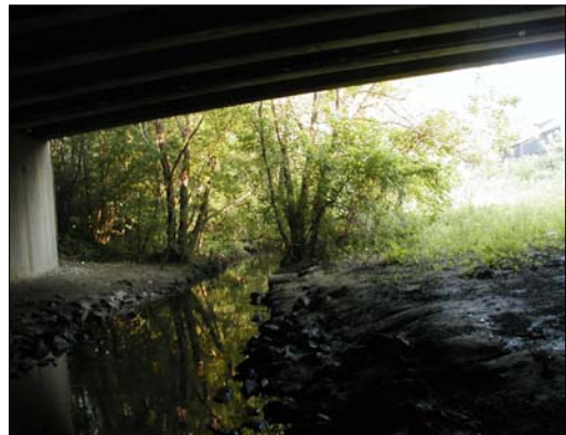
H15: Black Creek facing upstream (north) from the Steeles Avenue bridge.
