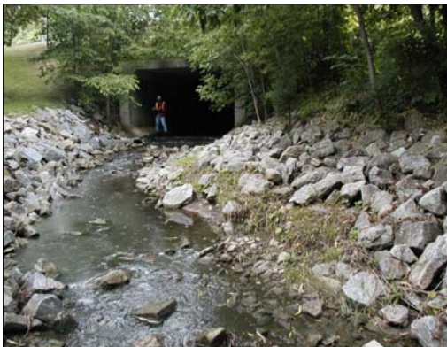
R9: Exhibition Creek facing upstream (north) towards the Highway 7 culvert.
