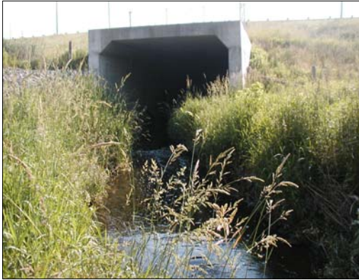
H13: Black Creek facing upstream (east) towards the Jane Street culvert.
