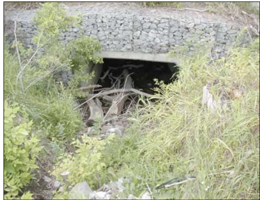
R4: Tributary of the Lower Rouge River, facing upstream (north) towards the Highway 7 culvert.
