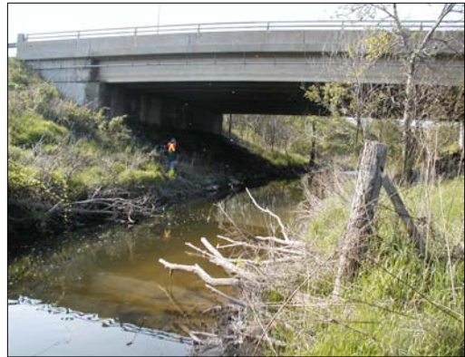
R3: The Upper Rouge River, facing downstream (south) towards the Highway 7 bridge.
