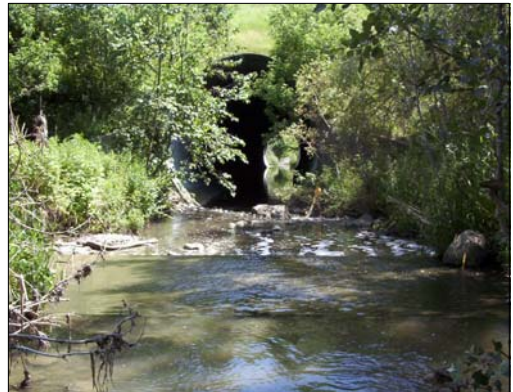
D12: German Mills Creek facing downstream (south) towards the Highway 7 culvert.
