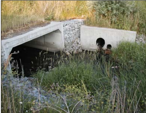
H12: Black Creek facing downstream (south) towards the Highway 7 culvert.
