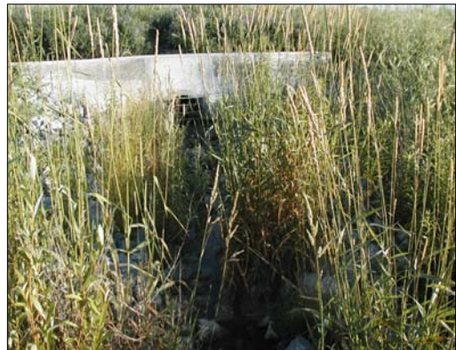
D18: Tributary of Westminister Creek facing upstream (north) towards the culvert, south of Highway 407.
