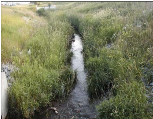
H12: Black Creek facing upstream (north) from the Highway 7 culvert.
