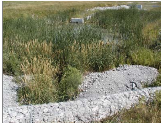
R11: Tributary of the Little Rouge River, facing R25 and upstream (north) from the Highway 7 culvert.
