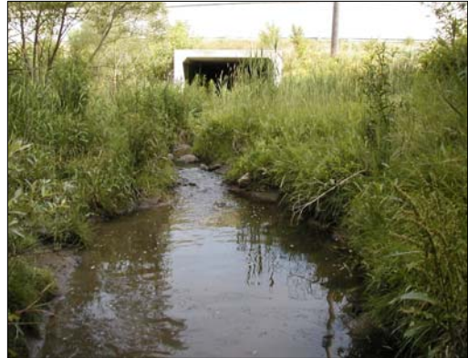
D9: Tributary of the East Don River, facing upstream (north) towards the Highway 407/Langstaff Road culvert.
