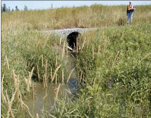
R11: Tributary of the Little Rouge River, facing upstream ( north) towards the Highway 7 culvert.
