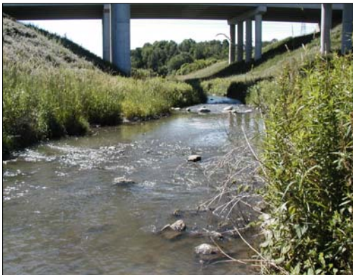
D7: The East Don River, facing railway bridge downstream (south) from the Highway 7 culvert.
