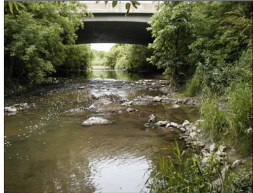
R5: The Lower Rouge River, facing upstream (south) towards the Highway 7 bridge.
