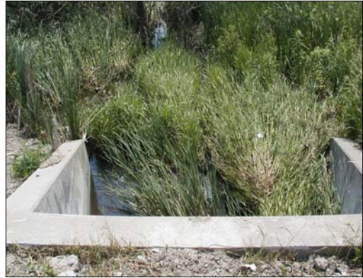
H6: Rainbow Creek, facing downstream (south) from the Highway 7 culvert.
