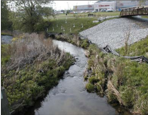
R2: Beaver Creek facing downstream (south) from the Highway 7 culvert.
