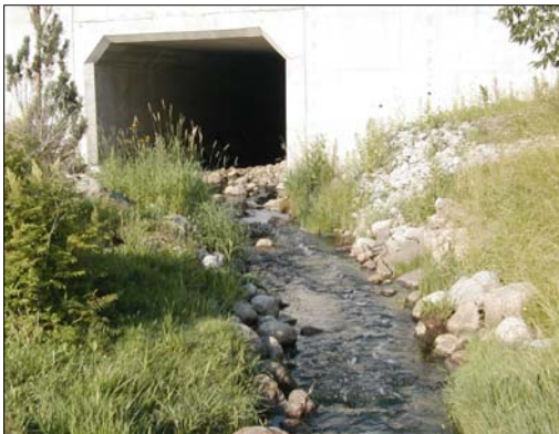
H13: Black Creek facing downstream (west) towards the Jane Street culvert.
