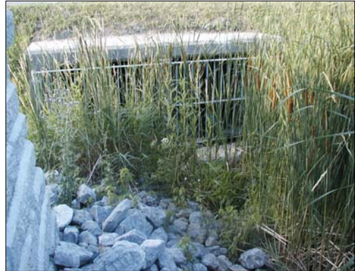
D19: Westminster Creek facing downstream (south) towards the Centre Street culvert.
