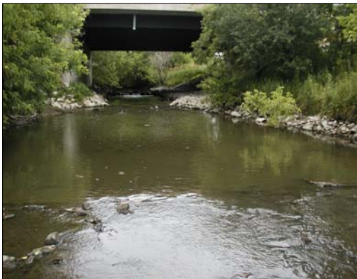
R6: The Lower Rouge River, facing upstream (north) towards the Highway 7 bridge.
