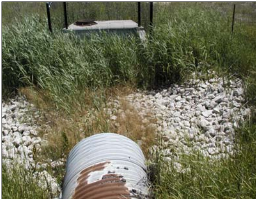
H3: Tributary of the Main Humber River, facing downstream (south) from the Highway 7 culvert.
