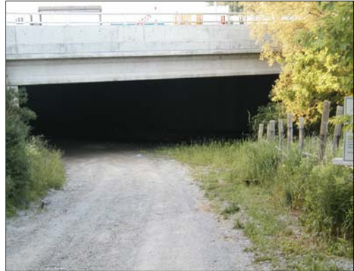
H15: Black Creek facing downstream (south) towards the Steeles Avenue bridge.
