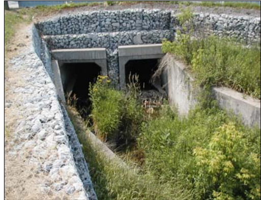
D1: Tributary of the West Don River, facing upstream (northwest) towards the Highway 7 culvert.
