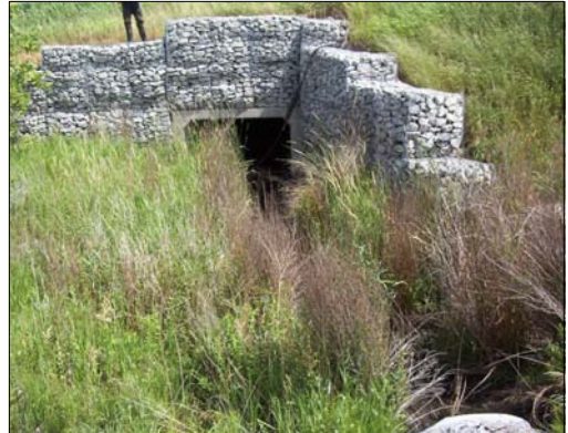
D14: Tributary of German Mills Creek, facing downstream (south) towards the Highway 7 culvert.
