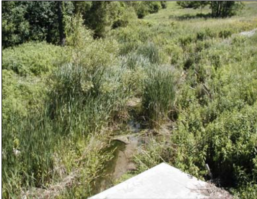
D22: Tributary of the East Don River, facing downstream (east) from the Bathurst Street culvert.
