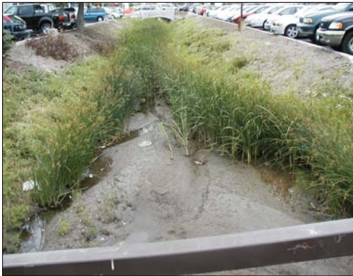
R22: Tributary of the Lower Rouge River, facing downstream (east) from the Main Street Unionville culvert.
