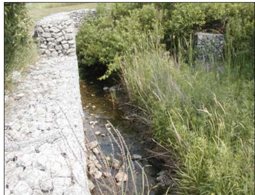
D1: Tributary of the West Don River, facing downstream (southeast) towards the Highway 7 culvert.
