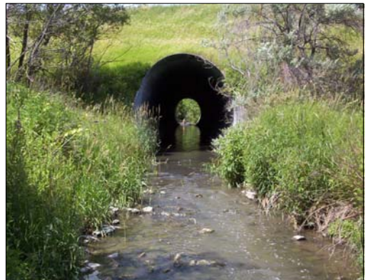
D12: German Mills Creek facing upstream (north) towards the Highway 7 culvert.
