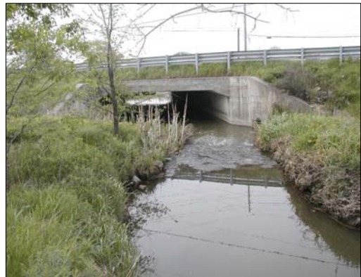
R2: Beaver Creek facing downstream (south) towards the Highway 7 culvert.
