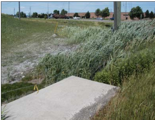
H4: Tributary of the Main Humber River, facing upstream (northeast) from the Highway 7 culvert.
