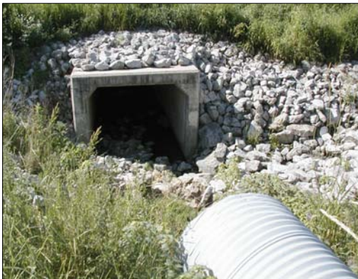
D6: Tributary of the East Don River, facing downstream (south) towards the Highway 7 culvert.
