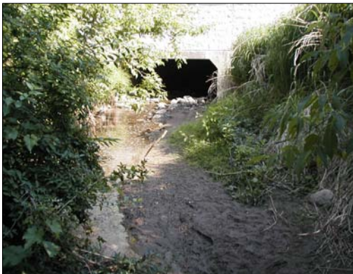
H8: Tributary of the Main Humber River, facing upstream (north) towards the Highway 7 culvert.
