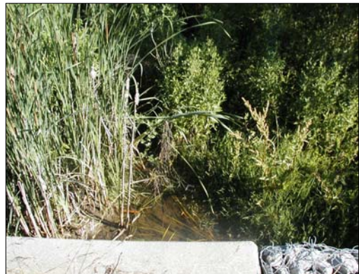
R10: Tributary of the Little Rouge River, facing upstream (north) from the Highway 7 culvert.
