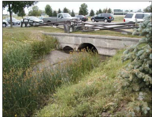
R22: Tributary of the Lower Rouge River, facing upstream (west) towards the Main Street Unionville culvert.
