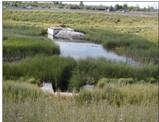
D6: Tributary of the East Don River, facing downstream (south) from the Highway 7 culvert.
