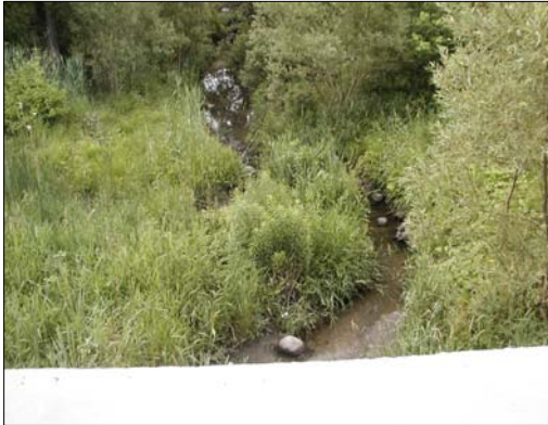
D9: Tributary of the East Don River, facing downstream (south) from the Highway 407/Langstaff Road culvert.
