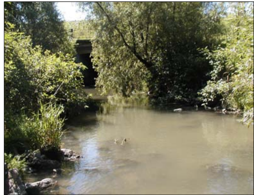
D7: The East Don River, facing downstream (south) towards the pedestrian bridge, with the Highway 7 culvert further downstream.
