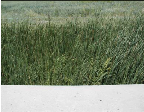
H1: Albion Creek, facing upstream (north) from the Highway 7 culvert.
