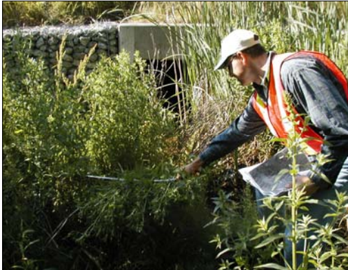
R10: Tributary of the Little Rouge River, facing downstream (south) towards the Highway 7 culvert.
