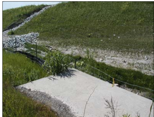
H4: Tributary of the Main Humber River, facing upstream (northwest) from the Highway 7 culvert.
