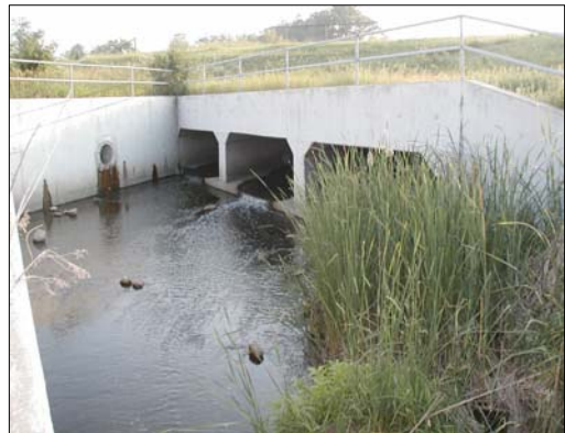
H12: Black Creek further upstream (north) from the Highway 7 culvert, at the stormwater management pond outflow.
