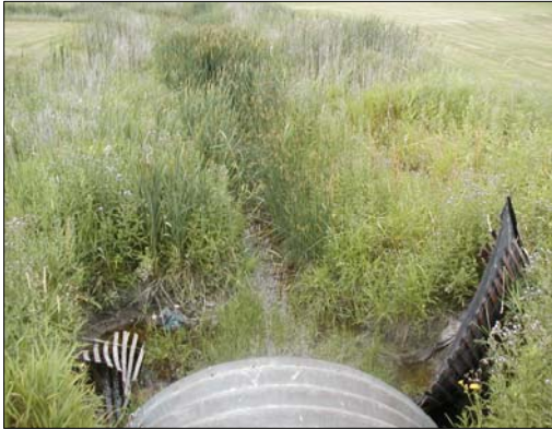
R22: Tributary of the Lower Rouge River, facing upstream (west) from the Main Street Unionville culvert.
