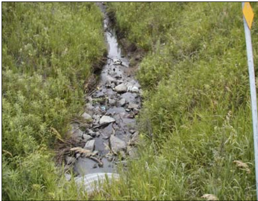
R1: Tributary of Beaver Creek, facing downstream (north) from the Highway 7 culvert.
