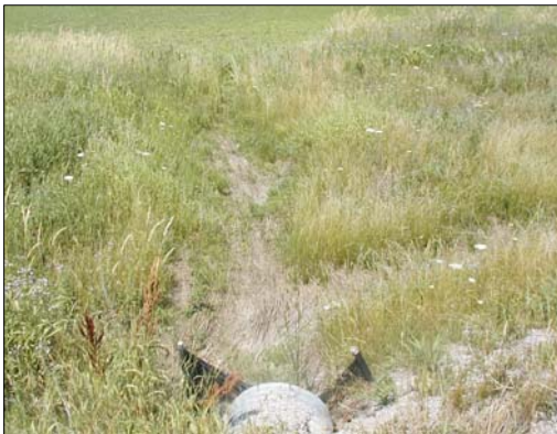
P2: Petticoat Creek, facing upstream (north) from the Highway 7 culvert.
