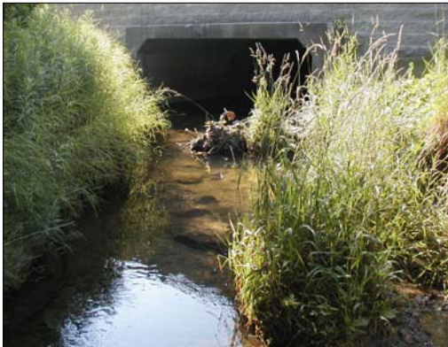
H8: Tributary of the Main Humber River, facing downstream (south) towards the Highway 7 culvert.
