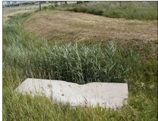
H4: Tributary of the Main Humber River, facing downstream (south) from the Highway 7 culvert.
