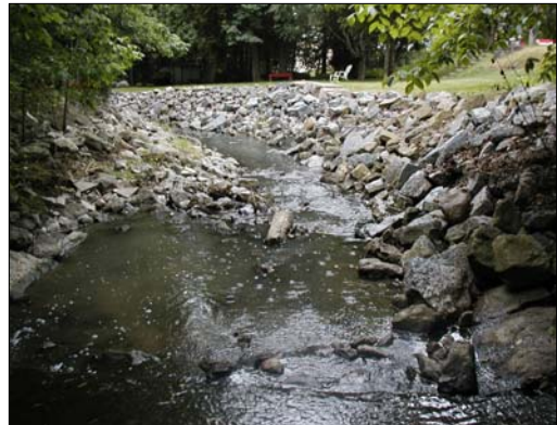
R9: Exhibition Creek facing downstream (south) from the Highway 7 culvert.
