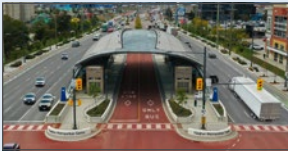
VMC BRT Station
