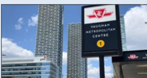
VMC Subway Station
